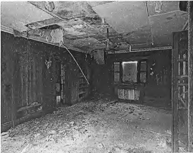
Mold and celing colapse
