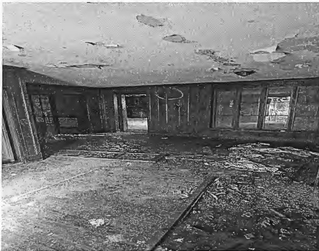
Floor & ceiling damaged by water intrusion
