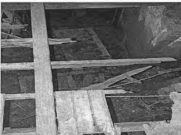
Severe floor damag
