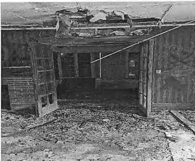
Mold & celing colapse
