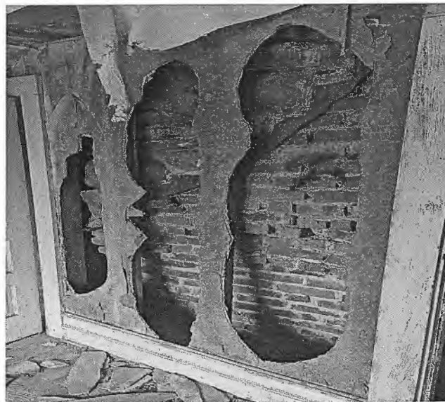
Deteriorated Fireplace
